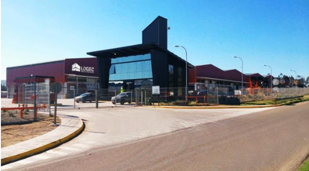
Logec warehouse entrance
