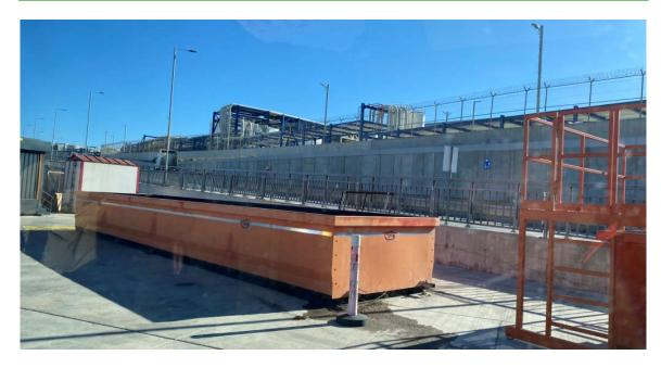
Photo 7: View of emergency secondary containment for potentially damaged containers.
