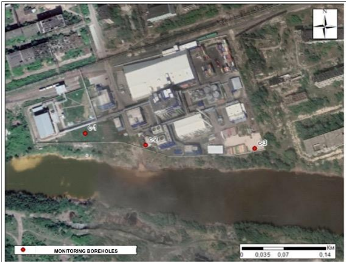
Figure 4: Location of Water Groundwater Monitoring Boreholes at Korund Zyan
